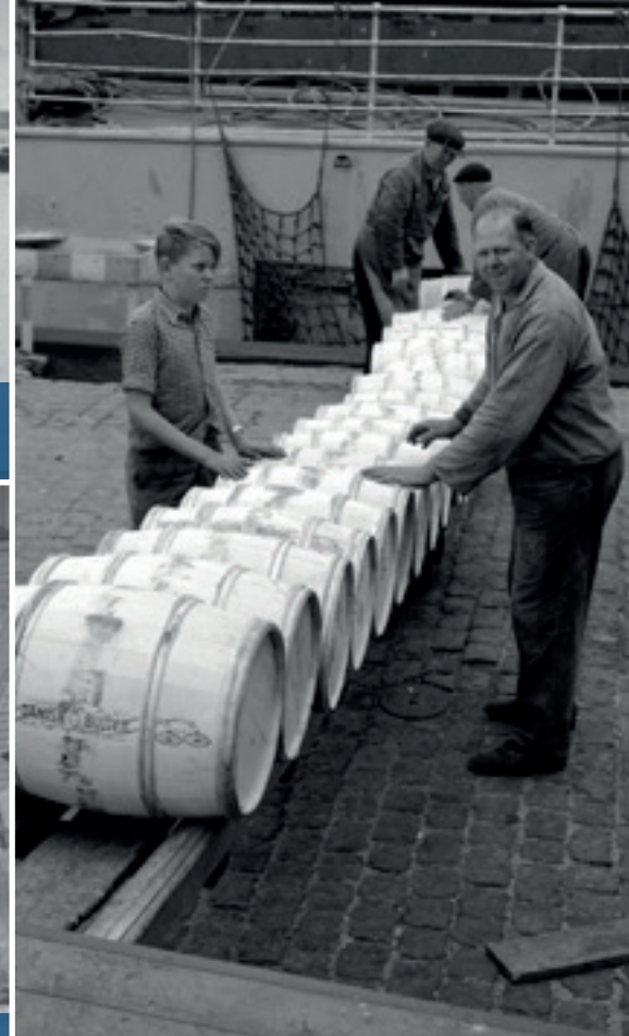
Loading of butter casks at East Port, in 1956. Note the safety net slung alongships to catch the casks if they tumble off the rolling ramp.
